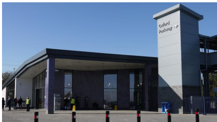
Oxford Parkway opened in 2015 and grew to serve over 1 million passengers in 2019.
