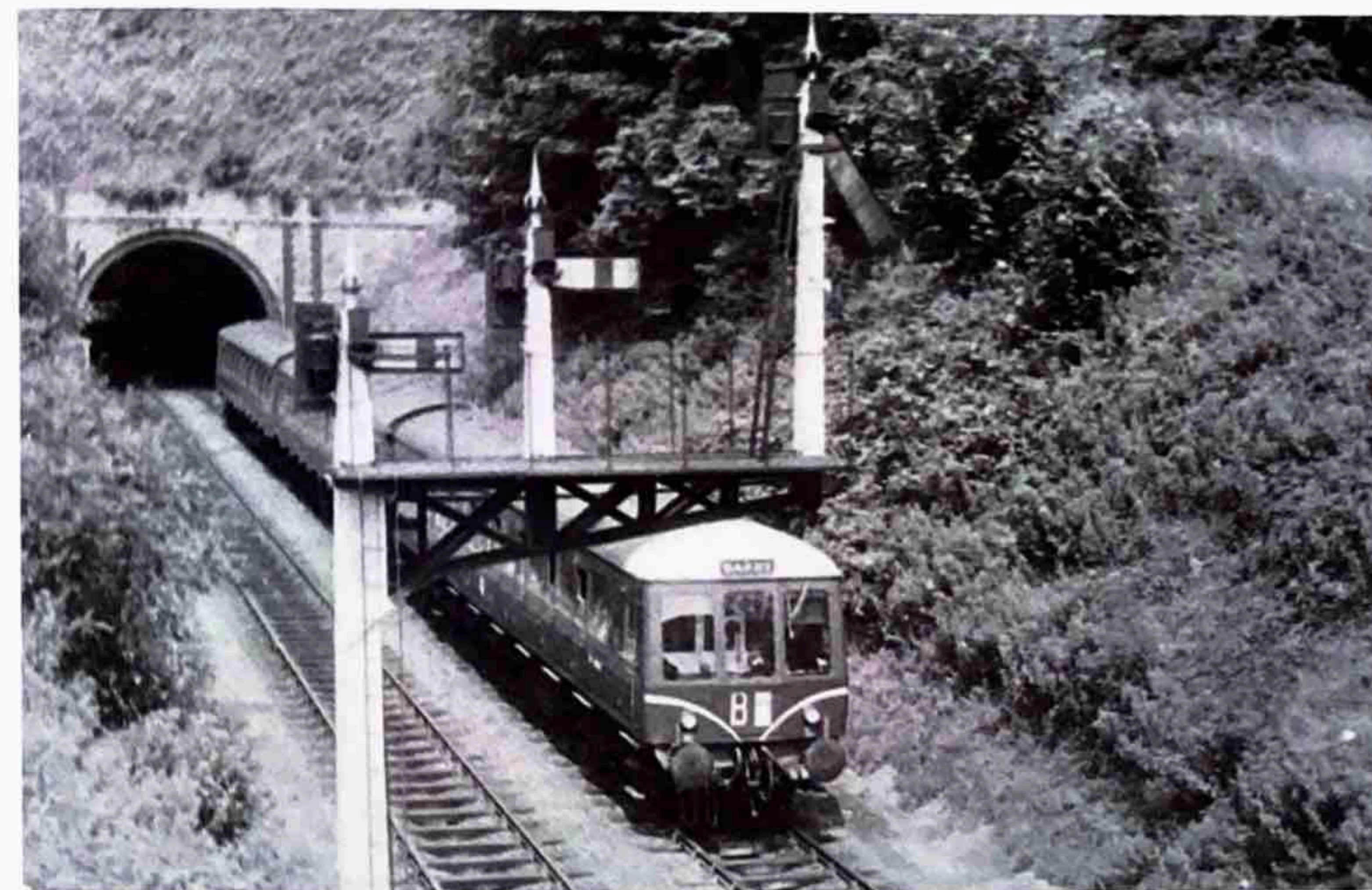
A 3 car DMU set (Class 116) emerges from number 1 tunnel bound for Barry with the 11.09 service from Bridgend on 25th July 1959. The tunnel is about 540 yards long.
