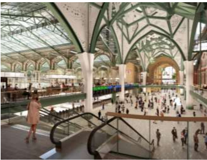
How the new concourse will look. The roof over the concourse will be removed, but the train shed over the platforms remains.
