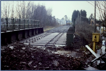
Figure 3 (left) . The railway underbridge with restricted 3.6 metre clearance over the A390 Callington Road at Gunnislake. The track seen on 5 th February 1994 has just been removed from it. Viewed towards Plymouth and closed Gunnislake station behind the camera. Figure 4 (right). The new station pictured on 23 rd July 1994 and taken from about the same view point. The railway underbridge has been removed and no longer obstructs the A390. Note the lower level of the railway. Pictures copyright of Roger Winnen - reproduced with permission.
