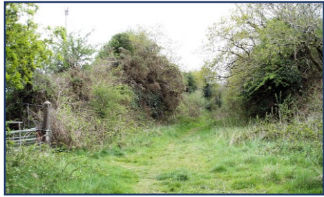
Figure 6. Descending on the 1 in 75 from the Abbotsfield bridge, this section of disused trackbed would be restored and regraded for the new station.
